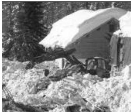
Figure 1: Clearing the Debris
