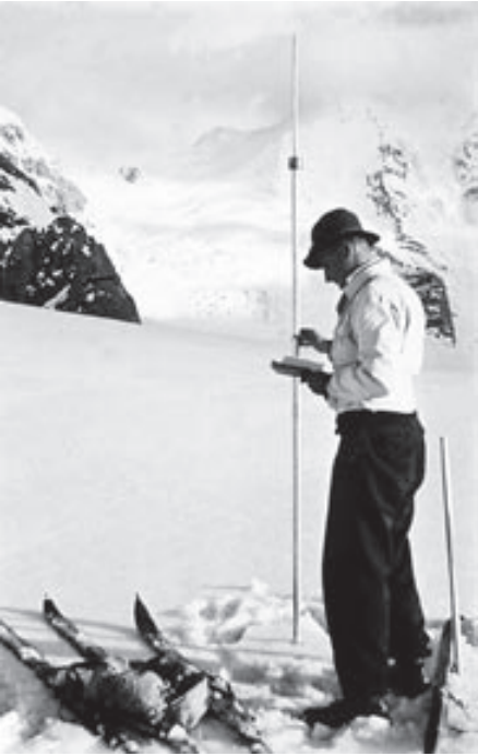
Measuring snow hardness with a rammsonde, 1937. Photo courtesy SLF archives
