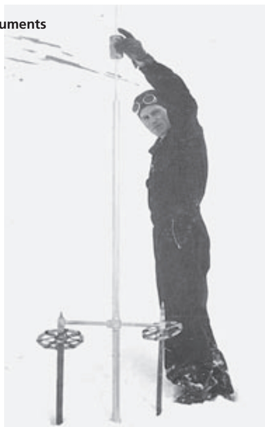
Cone penetrometer for measuring ram resistance.
