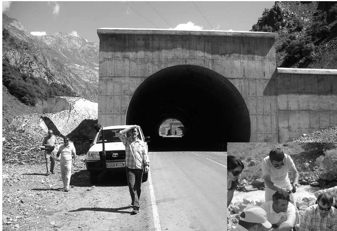
Left: Newly built tunnels protect a main road from one of the most obvious avalanche paths in Dunshabe, Tajikistan.
