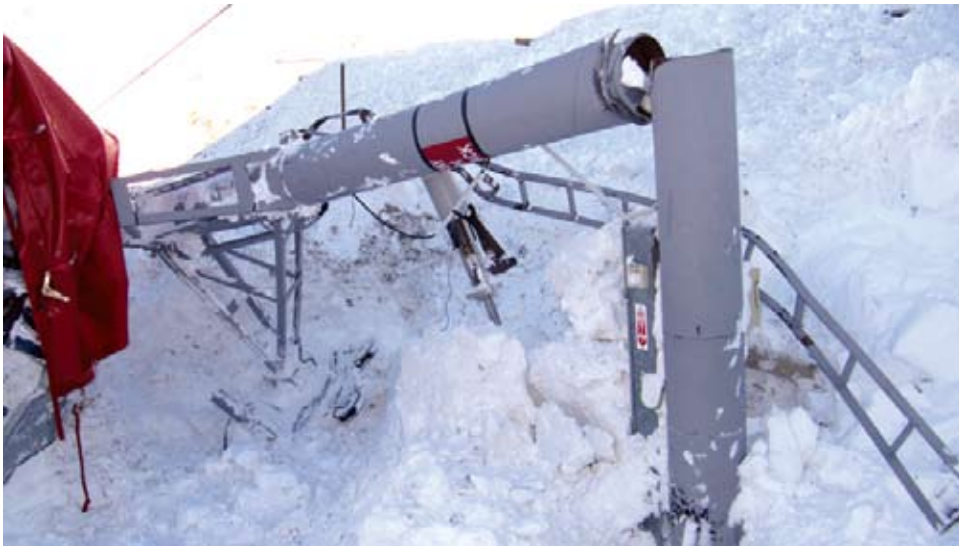
Avalanche-destroyed tower on T-Bar 1, Porters ski area. This break was not along a weld; ~3/8" steel snapped from the air blast and subsequent debris. Photo by Luke Armstrong
