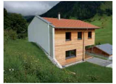
Residential building in a blue zone with structural reinforcement. The structural reinforcement increases the cost of a building by around 10%.
