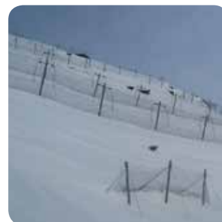
Dual protection wire net snow & rock fences
