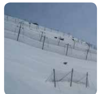
Dual protection wire net snow & rock fences
