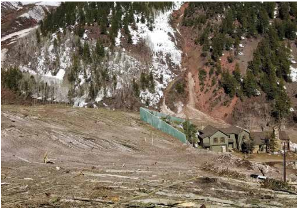
This concrete splitting wedge avalanche diversion structure designed by Art Mears saved this home in the Conundrum Creek valley south of Aspen.
